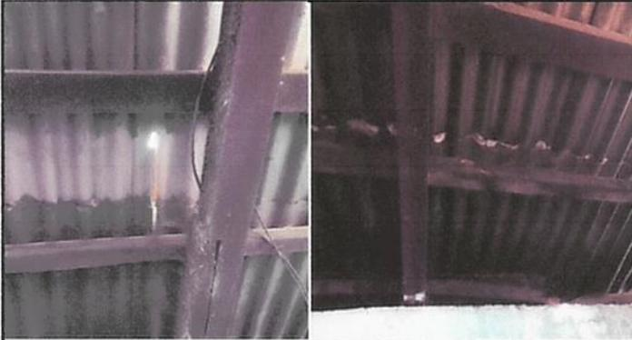
FOTO 1: TECHO CON LÁMINA EN MAL ESTADO Y ESTRUCTURA CON MADERA DETERIORADA
